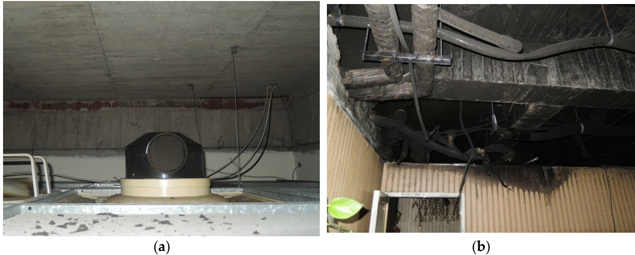
Figure 4. (a) The wall is connected to the floor structure above (a real photo of the scene, but not an institution mentioned in this paper). (b) The wall is not connected to the floor structure above (a real photo of the scene, but not an institution mentioned in this paper).
